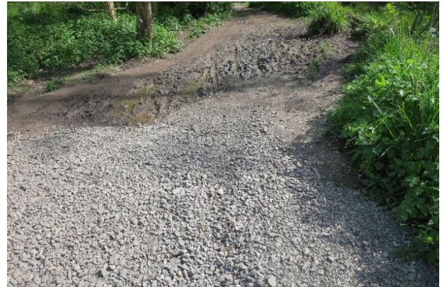
Here the work stopped.
