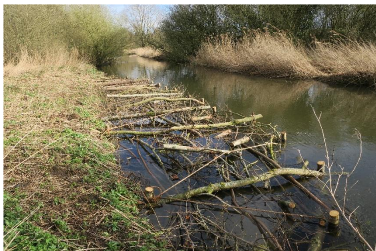
Newly constructed woody berm
