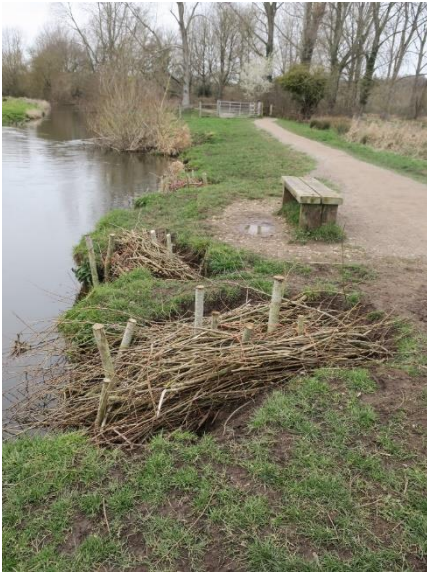
Bank reinforcement on Marston Marsh
